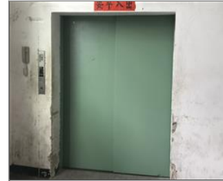
Photo of the inside of the main production hall 88 Cargo lift.JPG
