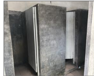
Photo of the sanitary facilities 132 Toilet.JPG
